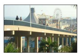
**Project Justification:** The Pier Bridge structural sufficiency rating is very low at 17 out of 100.
